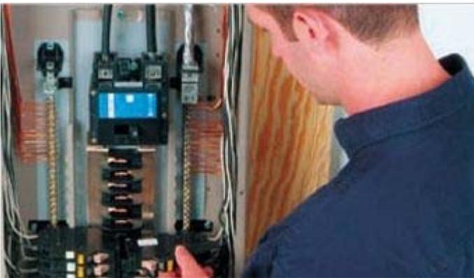
Generally used in loadcenters, panelboards, or similar device for electrical circuit protection, circuit breakers are available for a wide range of applications. The addition of Arc-Fault Circuit Interrupters (AFCI) represents a major improvement in electrical fire safety. Innovative safety device designed to prevent death and destruction caused by electrical fires.
